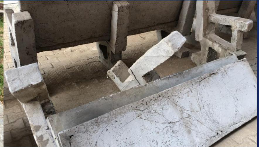
These were more heavily built than the previous two. Three supports instead of two. Yet, the failures were more dramatic: DOA: Some were already failed structures even before the buildings of the DLI were commissioned!
