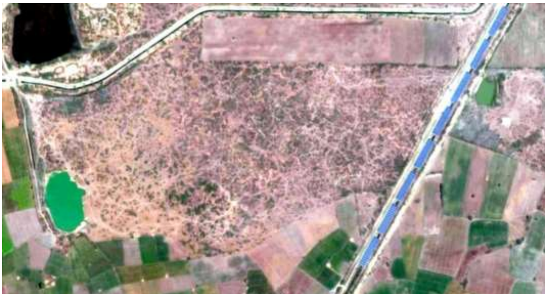
Figure 4. Canal Solar PV in India
